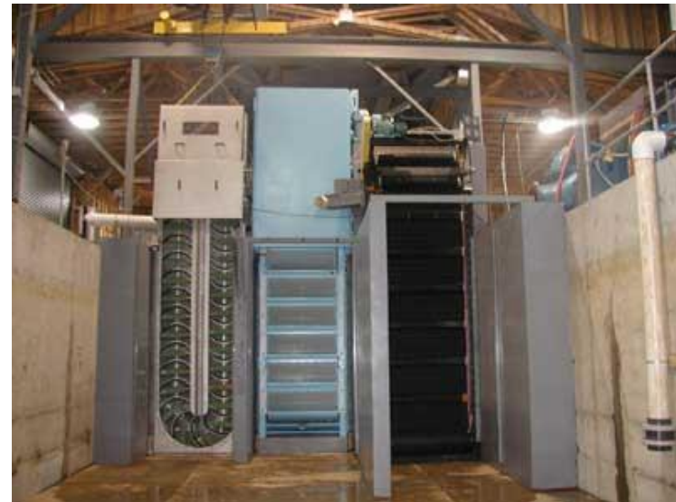
Parallelversuch versch. mech. Barrieren EPRI/ Alden Research Laboratory ( www.power-eng.com )
